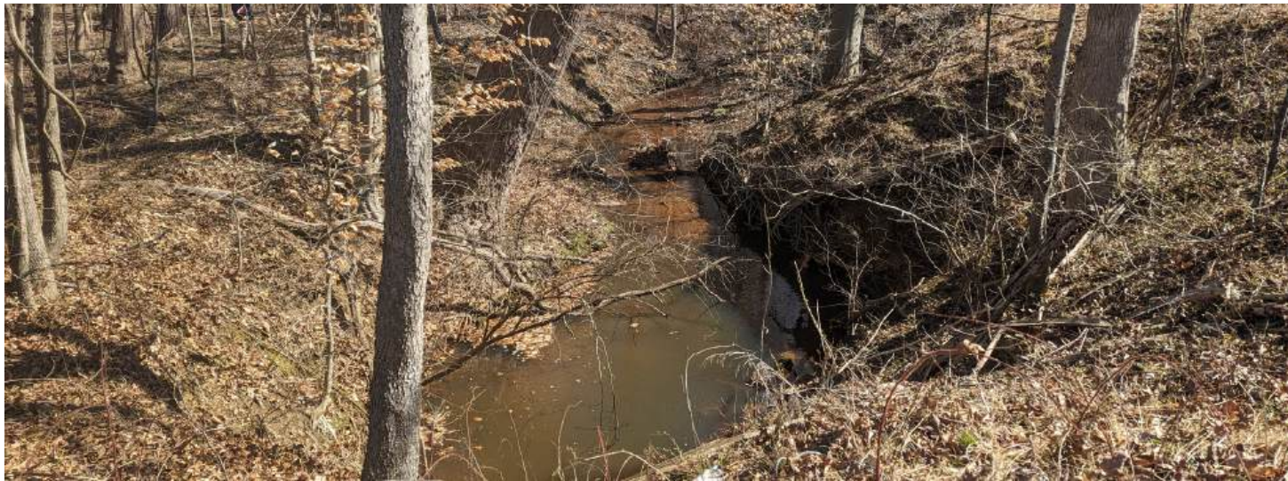
FIGURE 14 Daylighted stream outflow from Lower Pond.
