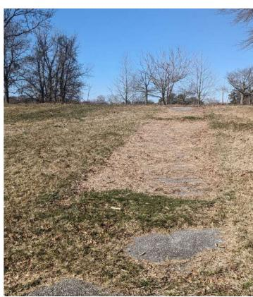
FIGURE 17 Sinkholes and failing pavement illustrate the poor condition of the existing cart path network.
