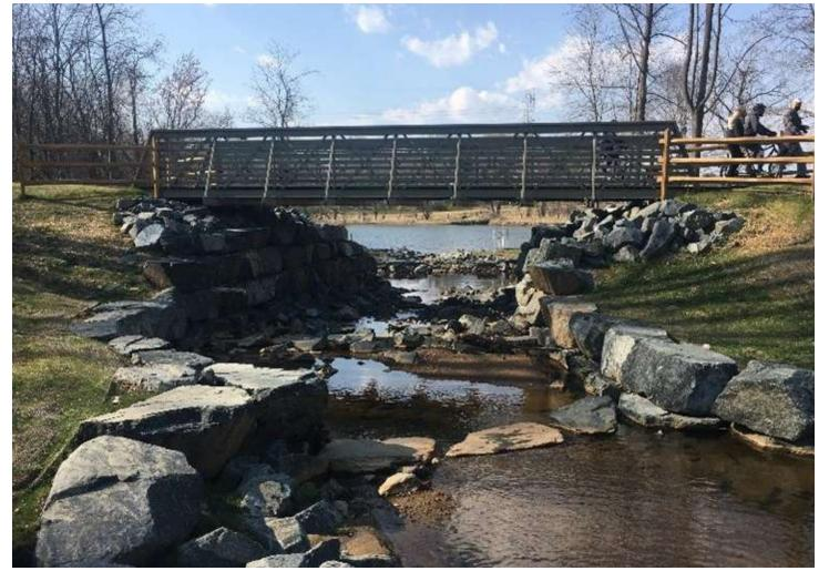
FIGURE 29 Example Stream Restoration with bridge and armored banks (Rustling Leaf stream restoration).
