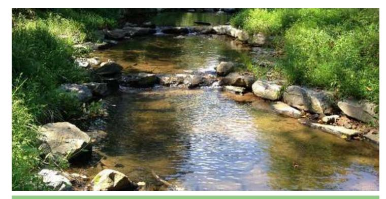
FIGURE 28 Example Stream Restoration with step-pools.
