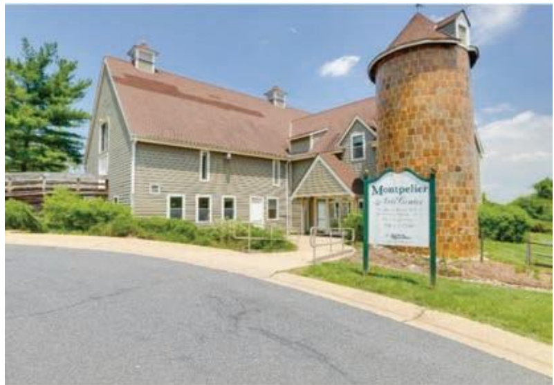
Montpelier Arts Center exterior
