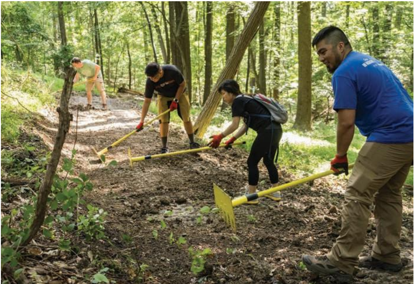
Volunteer trail construction at Fairland Recreational Park
