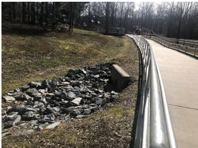
Stormdrain pipe passes under accessible route
