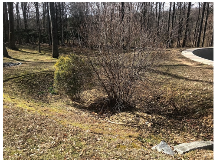
Micro-bioretention feature adjacent to skatepark
