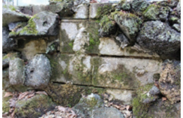
Deterioration of the mortar and stone
