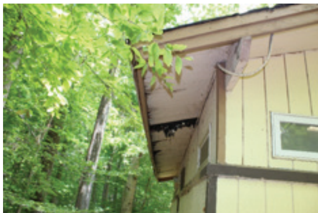
Hole in the roof
