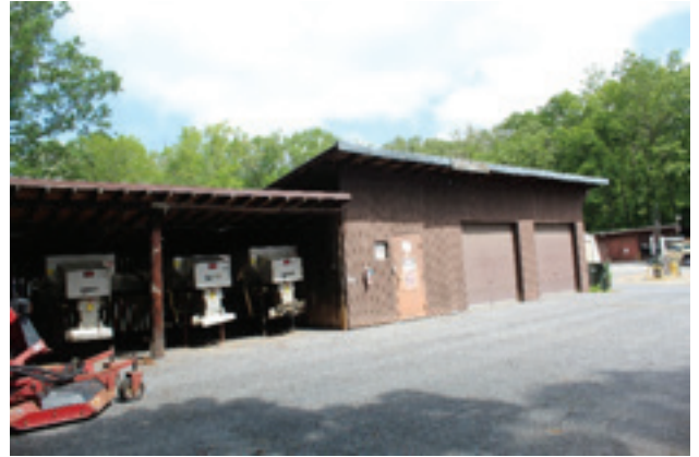
Open storage with deteriorated roof structure
