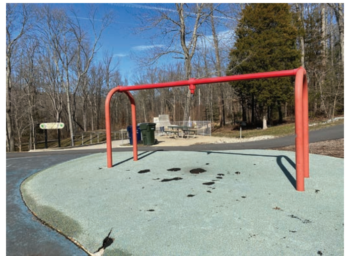
Play structure with missing equipment and torn rubber surfacing at upper playground
