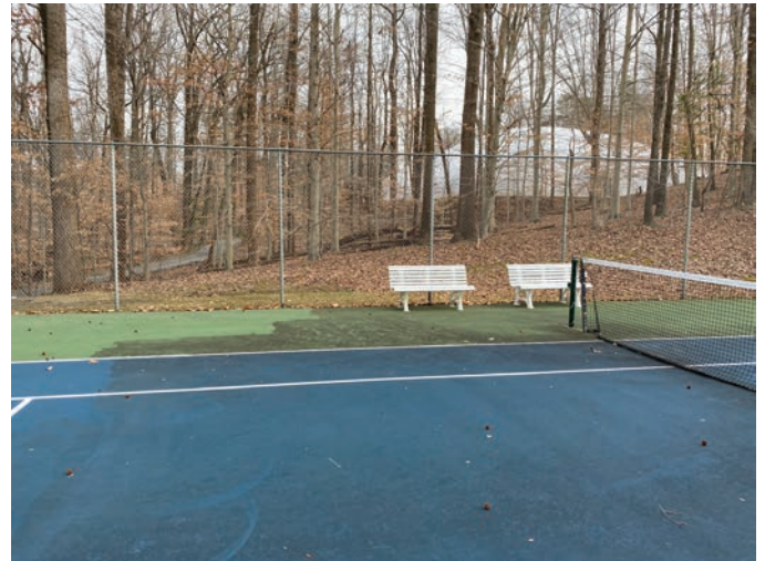
Water damage is visible on the court surface
