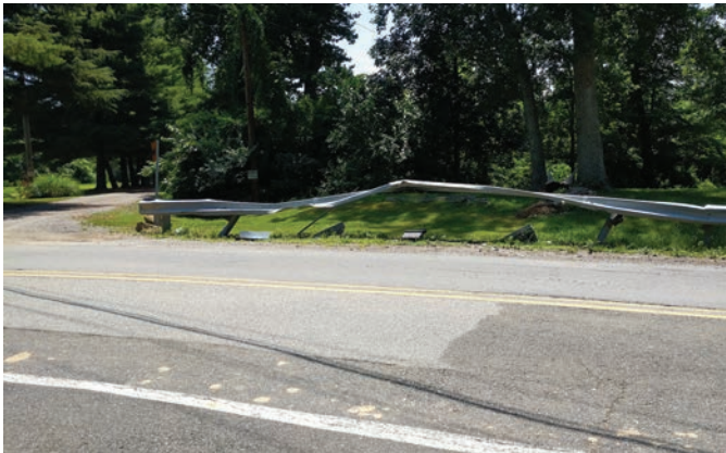
Damaged guardrail across Tippet Road from Schoolhouse, Wyoming Farm driveway on left side of image
