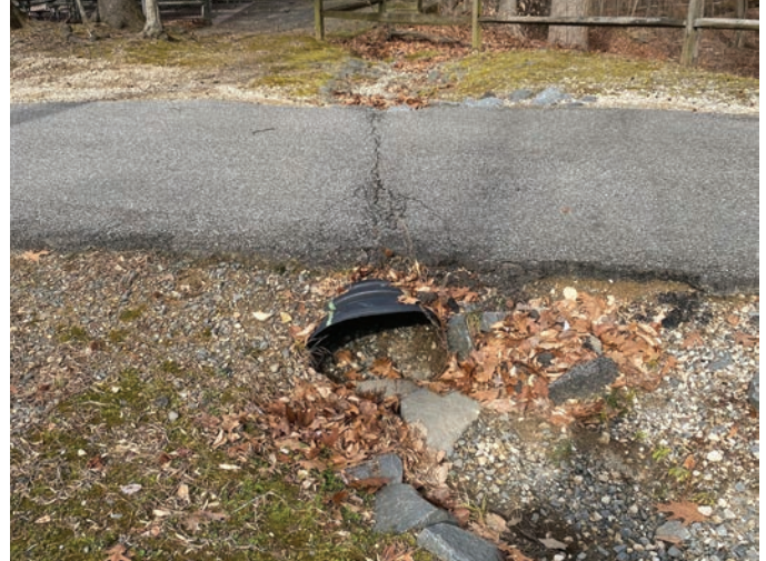
Damaged corrugated plastic pipe located near shelter 6
