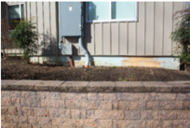
Staining on the foundation
