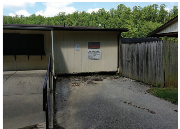
The boathouse, with stormwater debris from flow under structure
